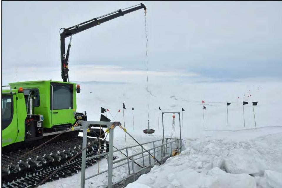
The new Scott Base tide gauge anchor being lowered into position on 3 November 2019
